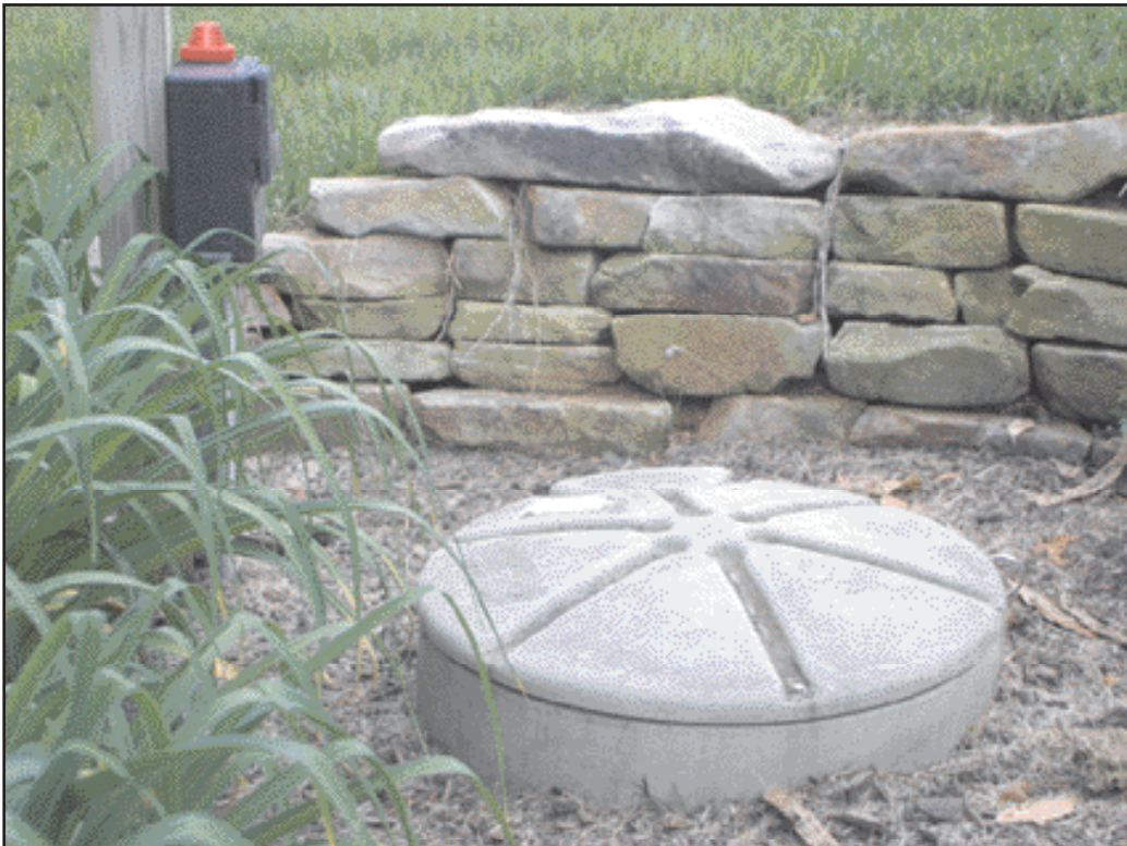
Low-pressure sewer pumps have a low-profile cover that blends into the landscaping yet provides easy access for servicing.
